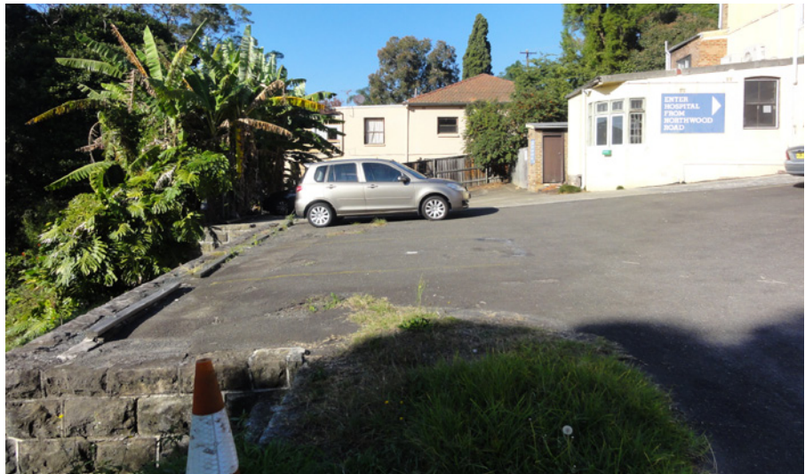
Rear surface car parking and retaining wall
