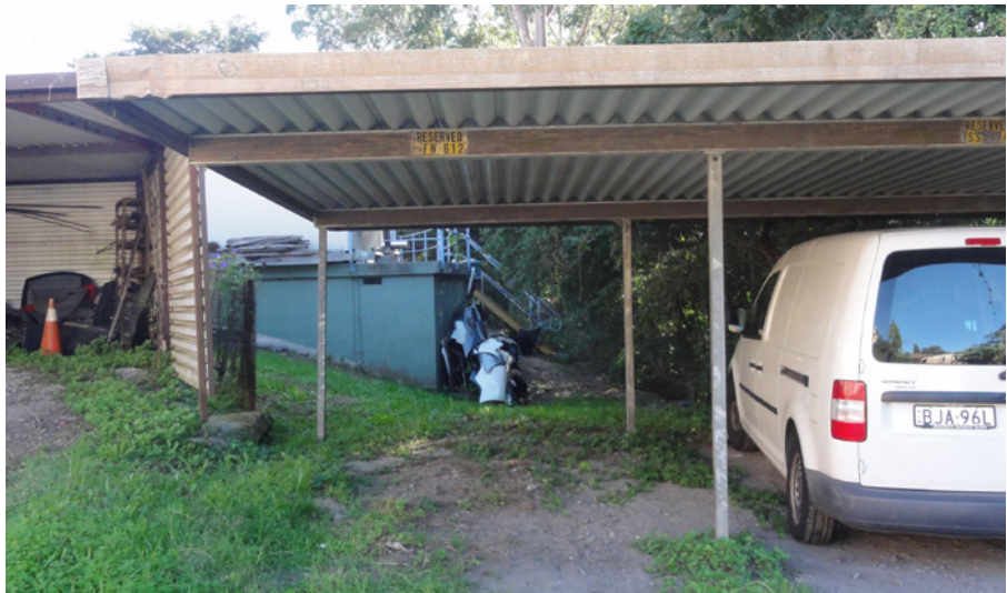
Existing structure and change of level at the rear boundary of the site
