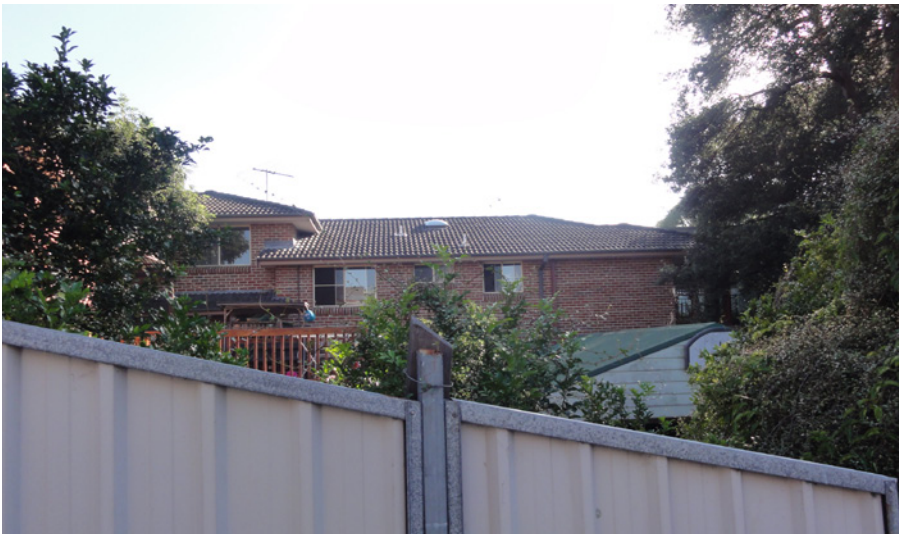
Existing residential flat building with habitable windows facing the northern boundary of the site
