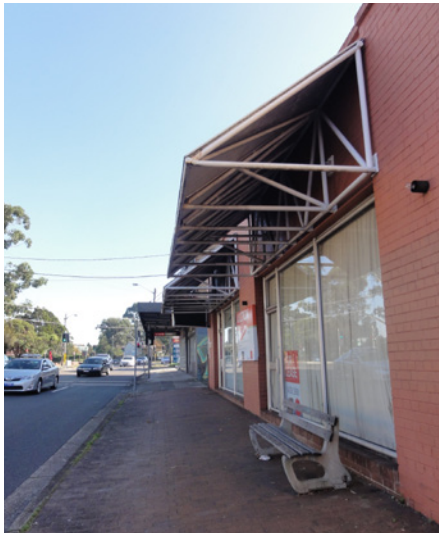
Existing poor amenity and inactive frontage
